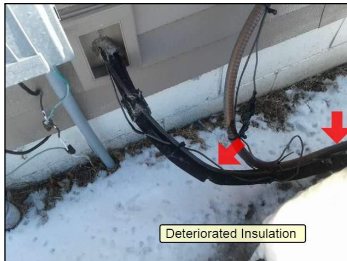
15. Insulation - missing
